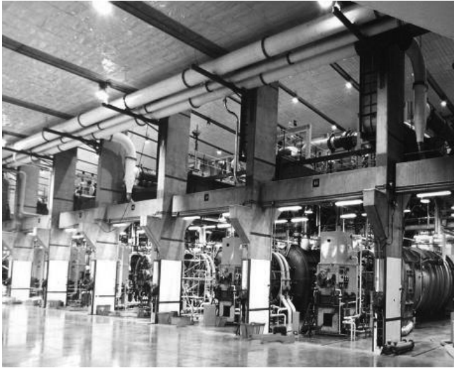
Figure 9-AI-1. View of the Enrichment Plant before Dismantlement. 9
